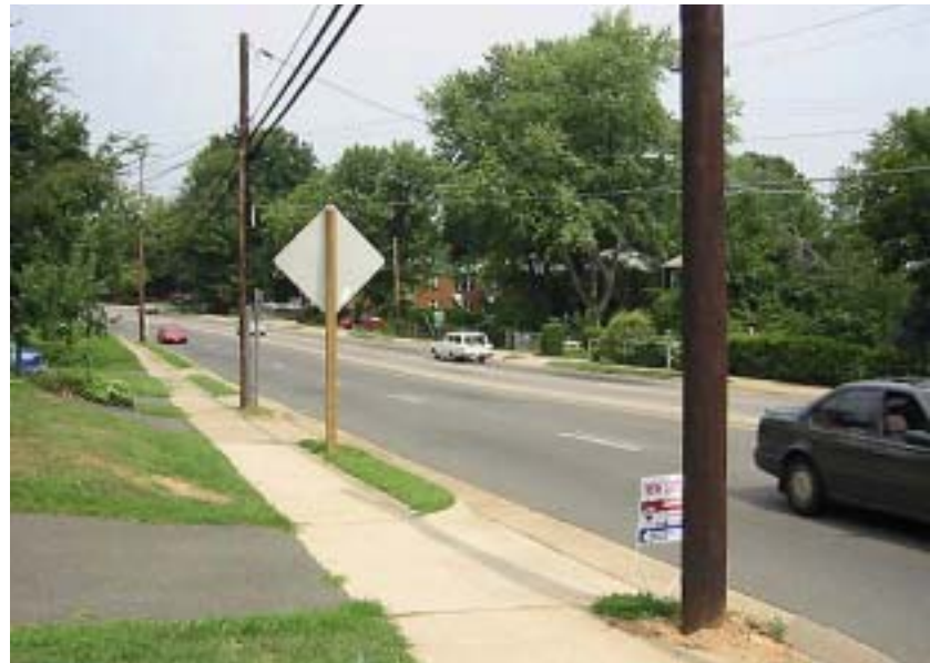
Narrow sidewalk close to four lanes of traffic on Huntington Avenue
